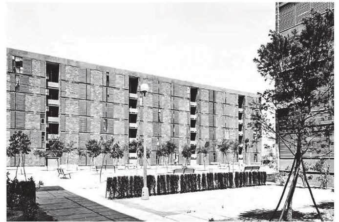
Figure 7: Block and semi-detached houses in the Sudoeste del Besòs estate
