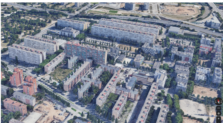
Figure 25: Semi-aerial photograph of the La Mina estate
