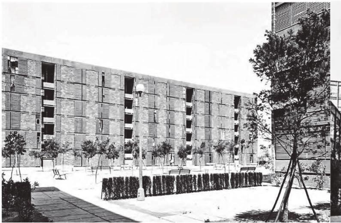
Figure 6: Blocks in the Sudoeste del Besòs estate
