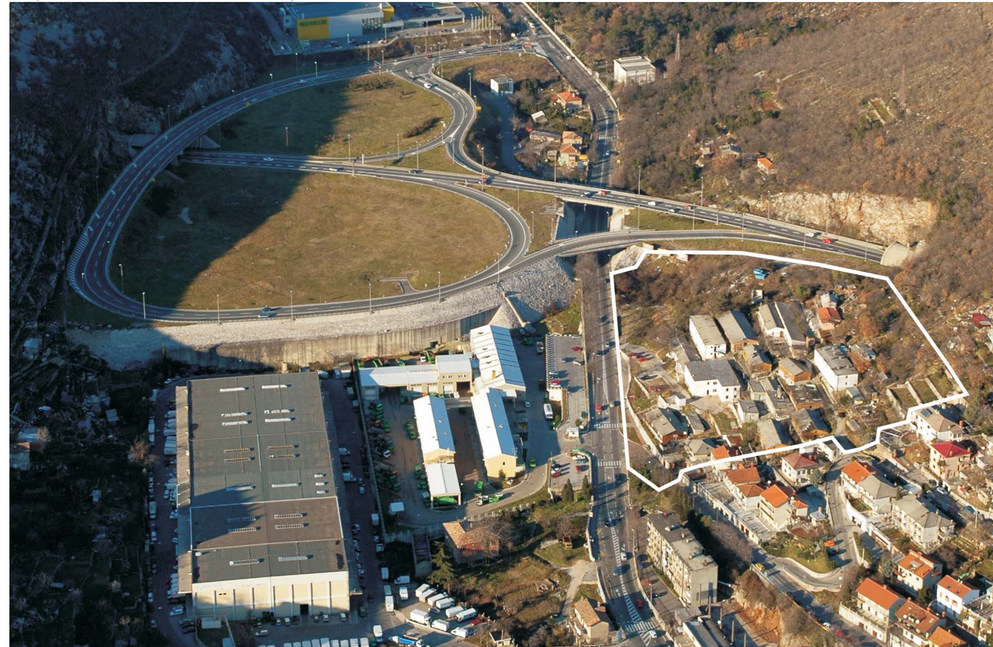
A - Areal view of the site
