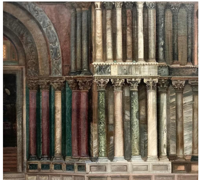
Facade detail of St. Mark Cathedral in Venice, which was partly built with reused columns or other decorative elements belonging to bizantine, egyptian or other buildings of the time.
