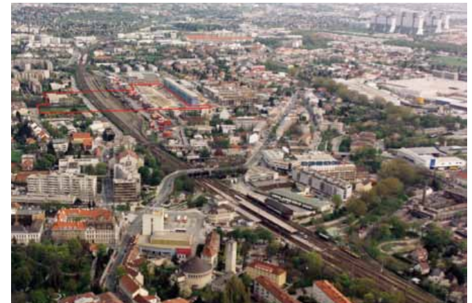
VIENNE E8 (AT) arch. Malarchitecture (NO) above: Liesing district
