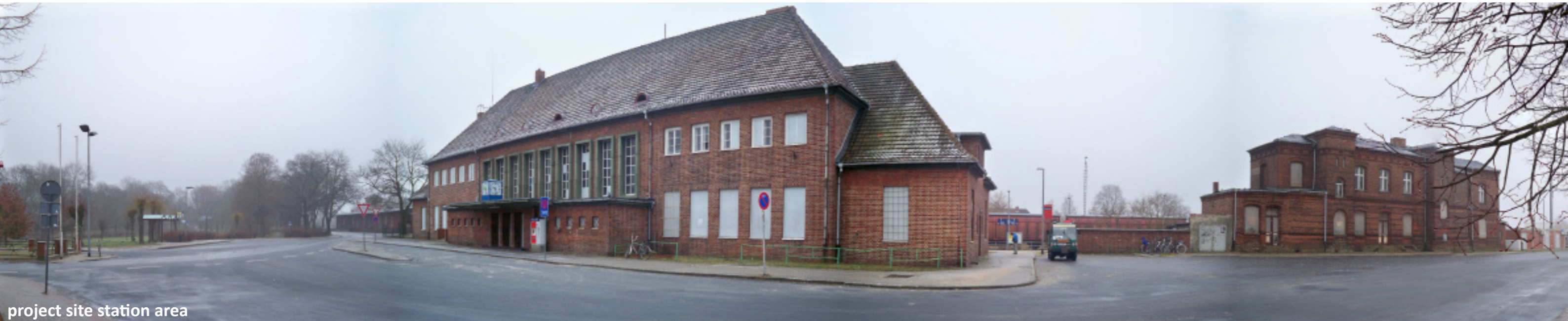
project site town entry Kyritzer Straße
