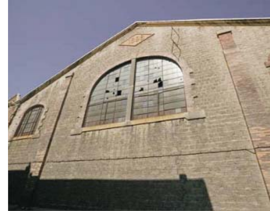
Gable of shed to be preserved
