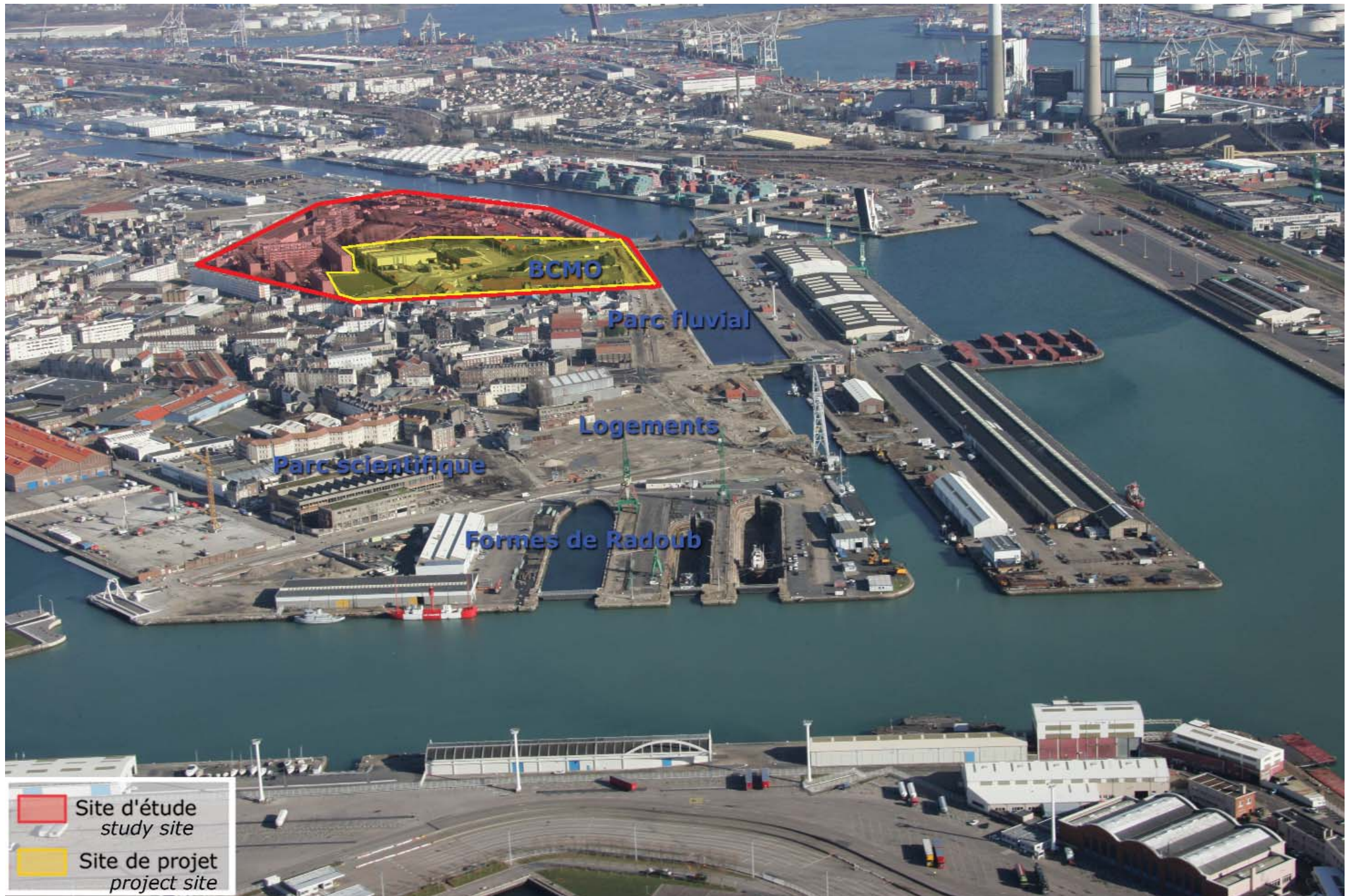
semi aerial photo of the site
