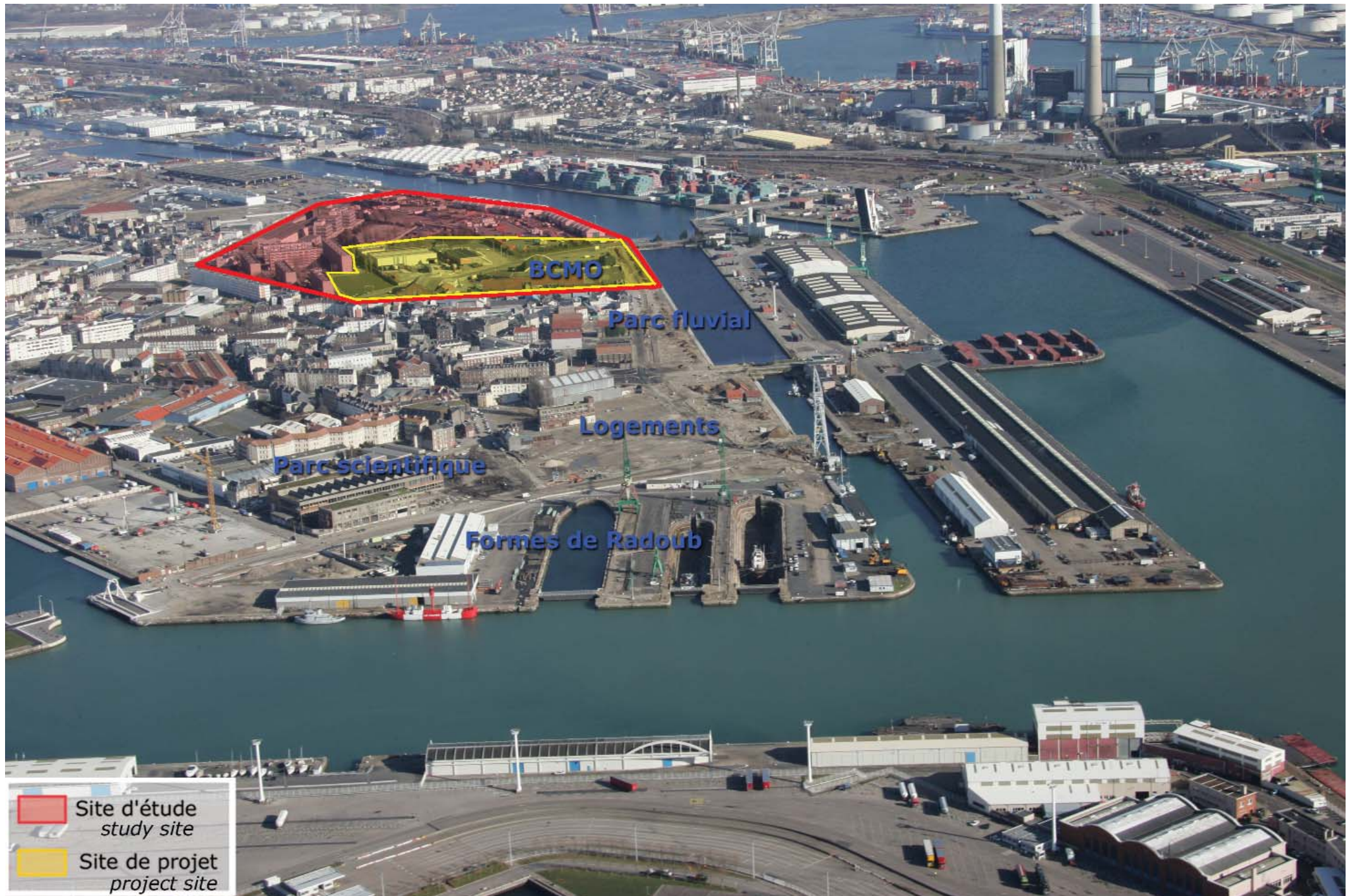
semi aerial photo of the site
