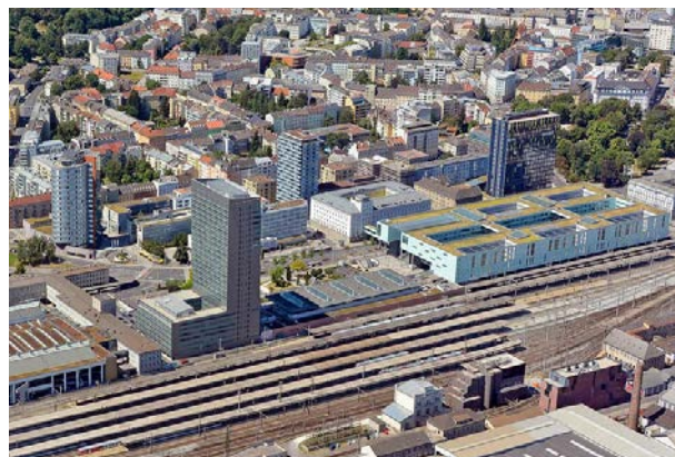
Aerial view station towards the north
