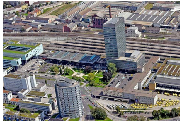
Main station with Terminal Tower, entrance and park
