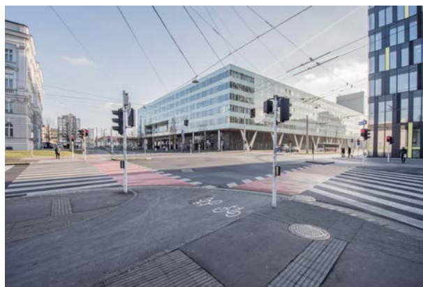
View from Volksgarten towards the site in the south; between ÖBB office left and the service centre in front
