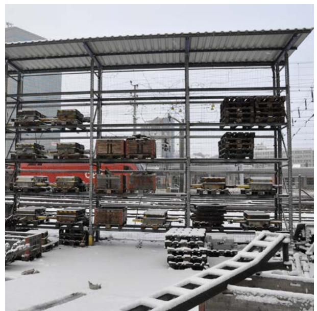
storage along the tracks
