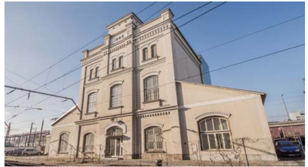
TS Werk, historical water tower, south of the tracks
