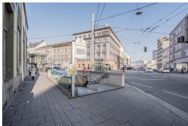
“Unionkreuzung”; access to underground station of the tram
