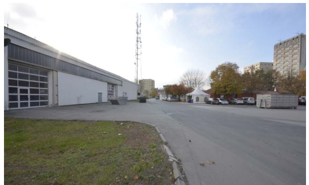
North facade Coca-Cola warehouse looking towards the bridge
