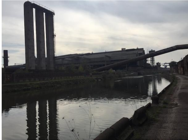
The towpaths were previously used to unload railway wagons. To facilitate unloading operations, the railway overhung the quays. The metal parts will be dismantled, while the concrete retaining walls will be maintained.
