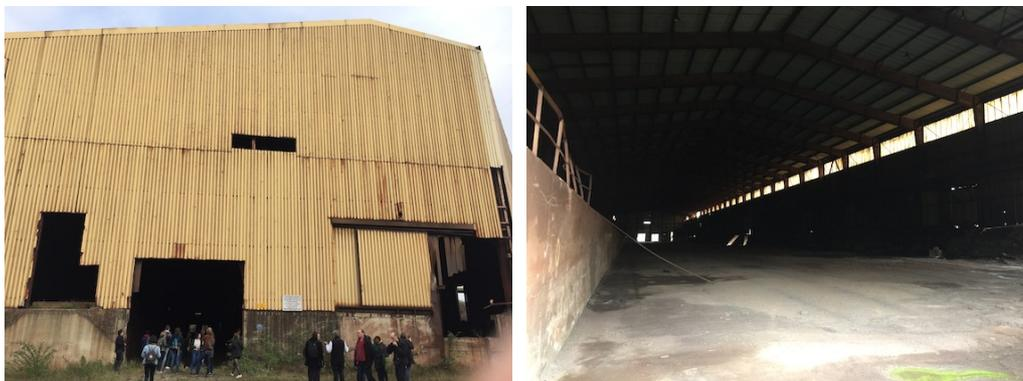
Going under the railway bridges, you reach a large building that runs along the road to Mons. Its surface area of 12,000 m<sup>2</sup> has the particular feature of having not intermediate support point, leaving a completely unobstructed space inside. This building can be maintained. Its structure is fit for purpose.
