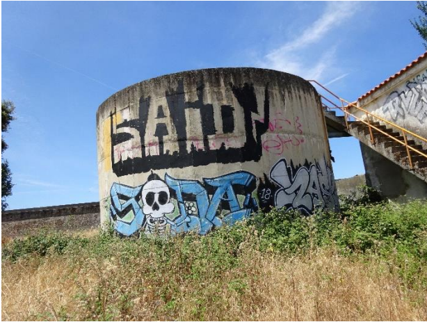
FORMER PANTANO DEL COJUGE FACILITIES
