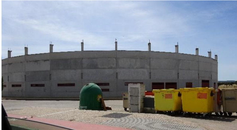
CASAR DE CÁCERES BULLRING_ACCESS FROM THE HOUSING DEVELOPMENT TO THE URBAN CENTRE
