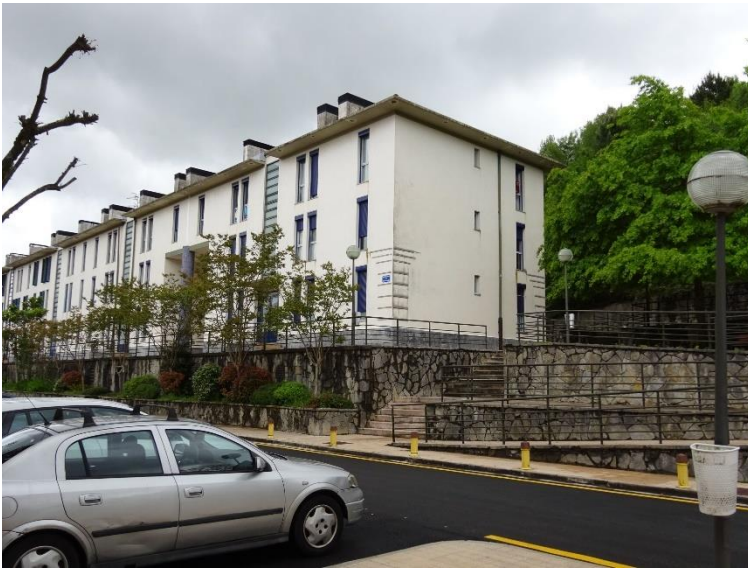
24. Social housing in Zelaialde district
