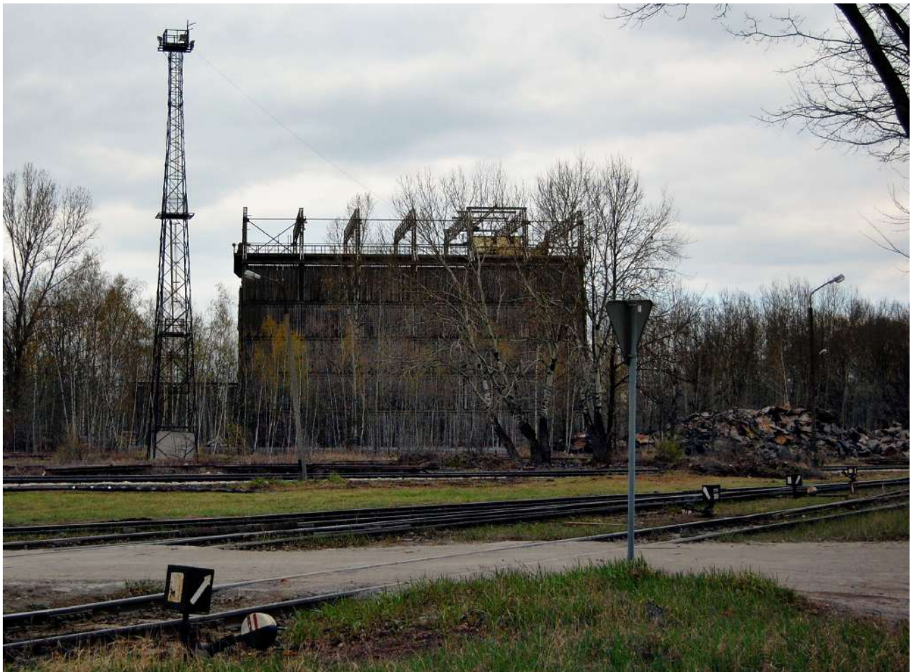
Pile driver hall
