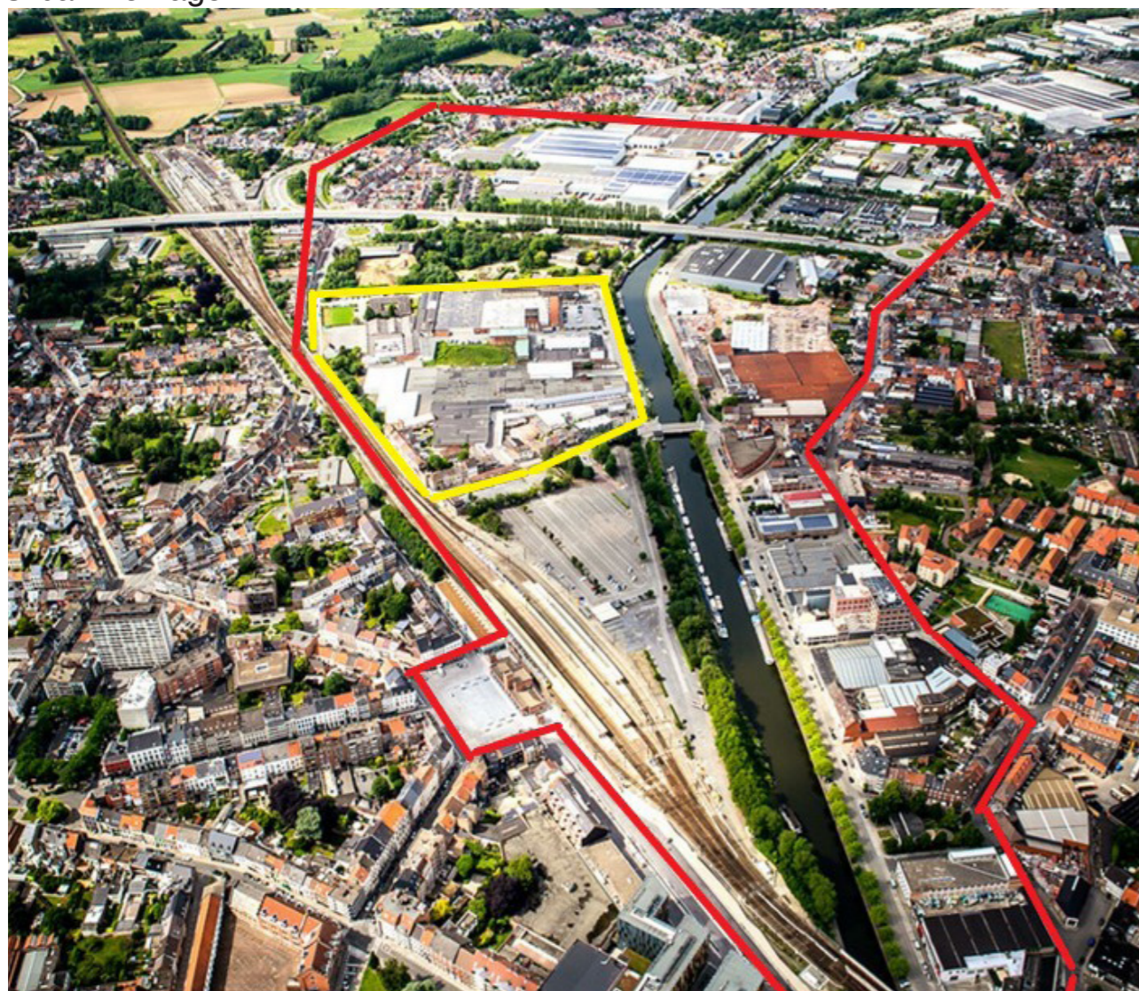
Oblique architectural view
