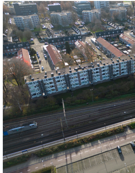
Aerial view P+R University Station
