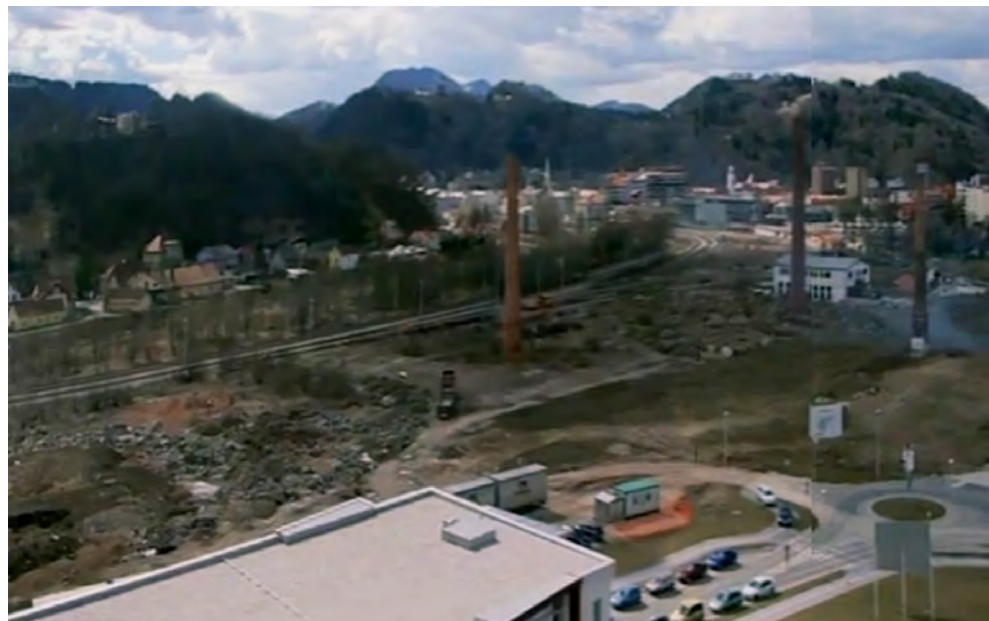
2009, After the demolition - landfill, © RTV documentary, 2009
