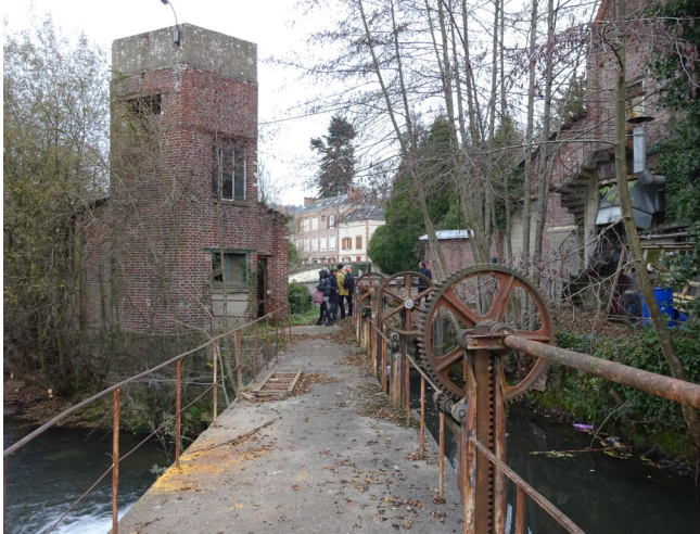
HYDRAULIC STRUCTURE, SIRET-DELAPORTE SITE, BRIONNE FR-INTERCOM_BERNAY_TERRES_NORMANDIE-PS1-P25
